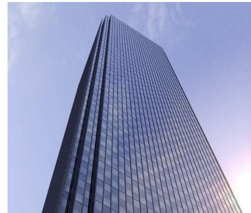
Semi-hidden Frame Curtain Wall (Vertical fixed Metal Component)
