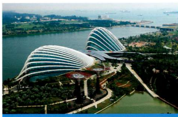
PROJECT: Gardens by the Bay ARCHITECT: Wilkinson Eyre, Grant Associates PRODUCT: 10YNE0175 +12A+6C+1.52PVB+6C (with firt) 6C+1.52PVB+6YNE0175 +12A+6C+1.52PVB+6C (with firt)
