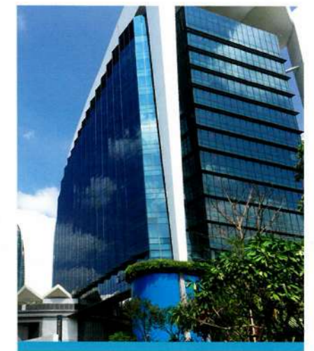
PROJECT: Howard Johnson Caexpo Plaza Nanning ARCHITECT: ECADI PRODUCT: 6C+1.14PVB+6C Low-E (4 # )+12A+6C
