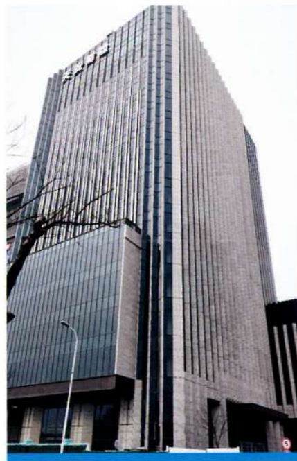
PROJECT: Shanghai Tian Financial Center ARCHITECT: Tongji Architectural Design Group Co.,LTD(TJAD) PRODUCT: 6C+1.52PVB+6 ultra high performance Low-E(4 # )+12A+8C
