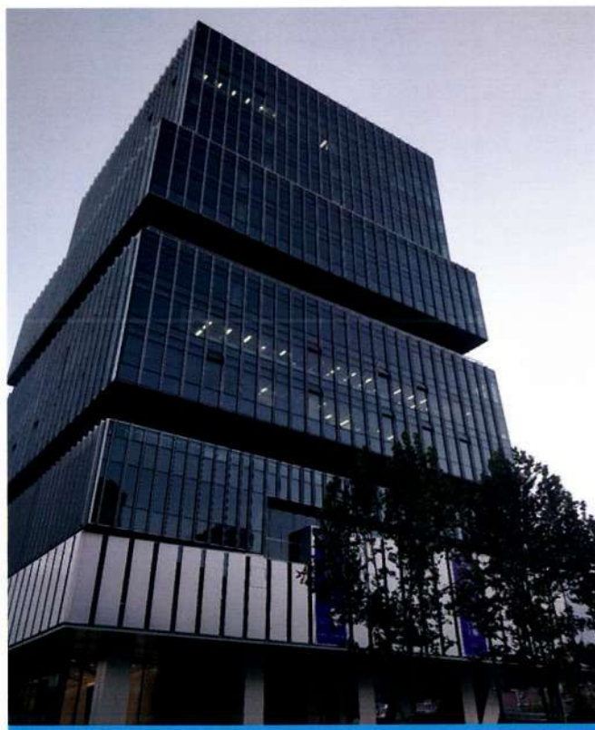
PROJECT: The Springs Center ARCHITECT: HenningLarsenArchitects (HLA) PRODUCT: 6C+1.14PVB+6YTE0155C (4 # ) +12A+8C 6C+1.14PVB+6YDF0148+12A+8C
