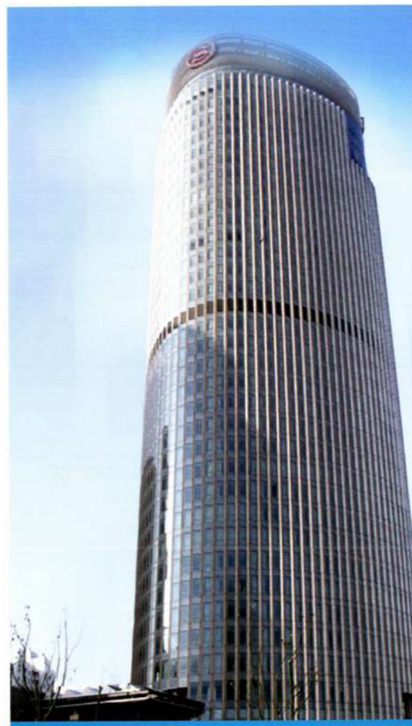
PROJECT: Shanghai Youyou Plaza ARCHITECT: B+H PRODUCT: 6SCLET0181(2 # ) frit+12A+6C 6SCLET0181(2 # )+12A+5C+0.38PVB+5C 8SCLET0181(2 # )Frit+12A+6C 6C(2 # )+12A+6C(4 # ) frit
