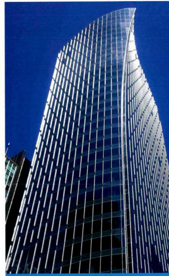
PROJECT: MNP Tower, Vancouver ARCHITECT: Kohn Pedersen Fox Associates (KPF) PRODUCT: 6YRE0146 (2 # ) +12Ar+6C
