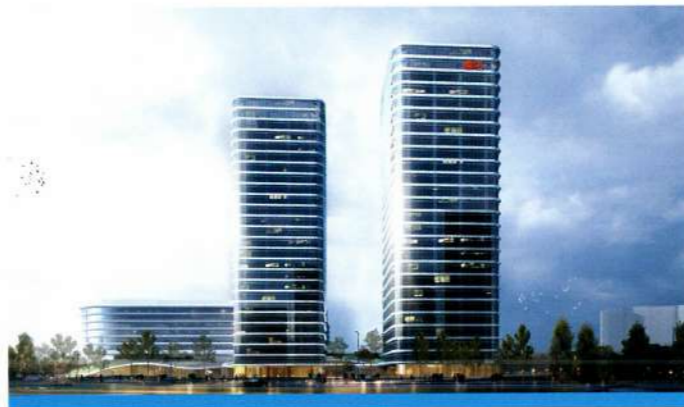
PROJECT: Xiamen Qudian Technology Financial innovation Park ARCHITECT: Ximen Baidi Jianzhu Sheji Youxian Gongsi PRODUCT: 5YSD0673 (2 # ) +1.52PVB+5YDT0648 (4 # ) +12A+6 Li 6YSD0673 (2 # ) +1.52PVB+6YDT0648 (4 # ) +12A+10 Li 6YSD0673 (2 # ) +2.28PVB+6YDT0648 (4 # ) +12A+10 Li(Bend) 10YSD0673 (2 # ) +1.9PVB+10YDT0648 (4 # ) +12A+12 Li 10YSD0673 (2 # )+2.28PVB+10YDT-0648 (4 # ) +12A+12 Li(Bend)
