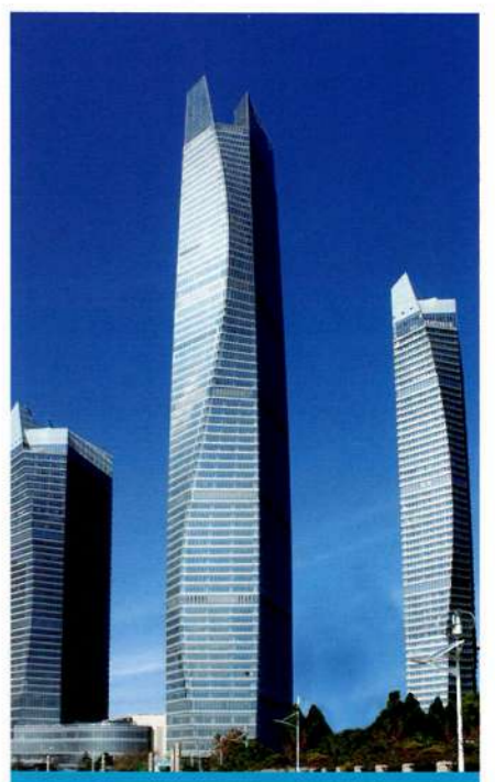
PROJECT: Qingdao Haitian hotel ARCHITECT: AA (Archilier Architecture) America PRODUCT: 8 Li+1.52PVB+8YKE0657T (4 # )+12A+8 Li 8 Li+1.52PVB+8YKE0657 (4 # )+12Ar+8 Li+12Ar+8Li
