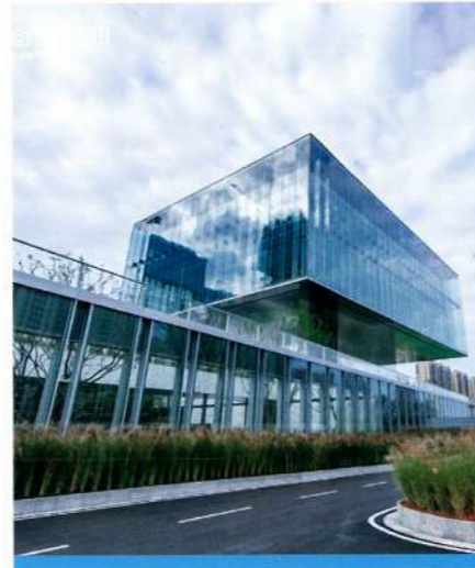
PROJECT: Sunac • Grand Milestone Modern Art Center Xi'an PRODUCT: 19+2.28SGP+19+2.28SGP +19+2.28SGP+19 all low iron glass
