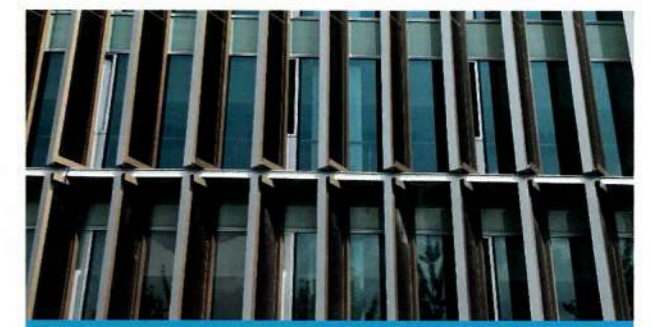
PROJECT: China Life Insurance Company Ltd.Data Center ARCHITECT: HENN-GmbH Germany PRODUCT: 6C+1.52PVB+3.2CIGS+1.52PVB+6C
