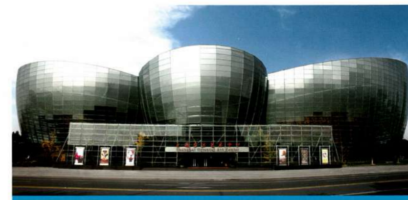
PROJECT: Shanghai Oriental Art Center ARCHITECT: Paul Andreu PRODUCT: 12C+1.52SGP+0.5Metal+1.52SGP+15C
