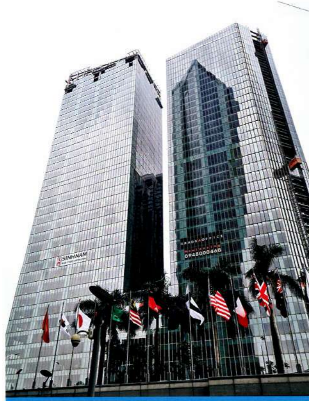
PROJECT: Metropolis Twin Tower ARCHITECT: Atkins Architects UK PRODUCT: 6C+1.52PVB+ 6YTE0145 (4 # ) +12Ar +8C
