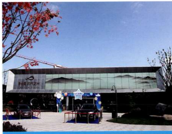
PROJECT: COUNTRY GARDEN Sales Office (Yibin) PRODUCT: 10C digital print frit (2 # ) +12Ar+10C LOW-E(3 # )
