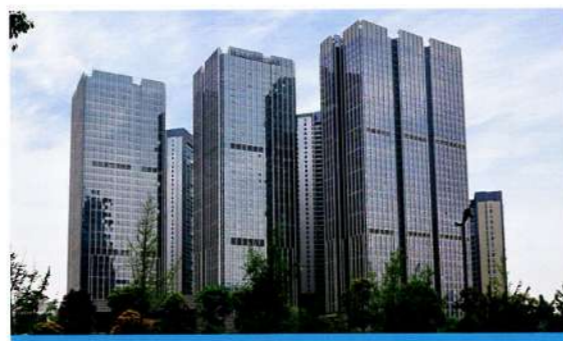
PROJECT: Forte Financial Center Chengdu China ARCHITECT: Hellmuth Obata Kassabaum (HOK) PRODUCT: 6C ultra high performance Low-E (2 # ) +12A+6C
