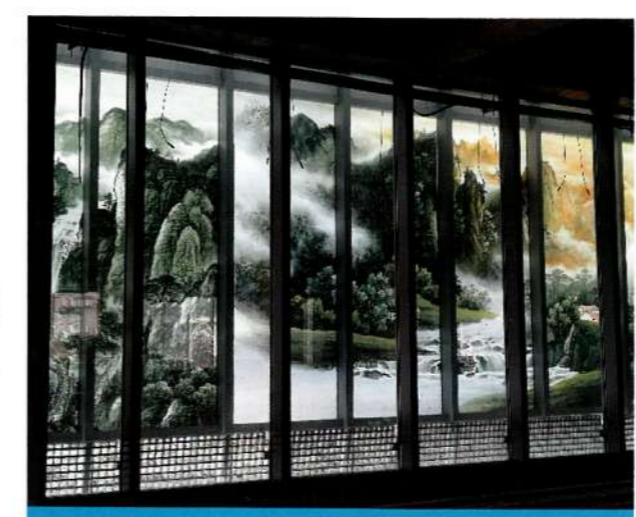
PROJECT: Cisen Pharmaceutical Co., Ltd. R&D Center ARCHITECT: SIGEE PRODUCT: 8 Li+1.52PVB+3.2CdTe+1.52PVB+8Li with digital print frit
