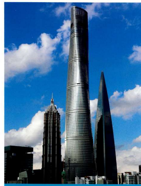
PROJECT: Shanghai Tower ARCHITECT: Gensler PRODUCT: External Skin(A): 12YSD0680(with frit)(2 # )+1.52SGP+12Li 12YSD0680(2 # )+1.52SGP+12 Li Internal Skin(B): 6 Li+0.89SGP+6YNE0659(frit)(4 # )+12A+8Li fire-proof 8YNE0659(2 # )+12A+8 Li
