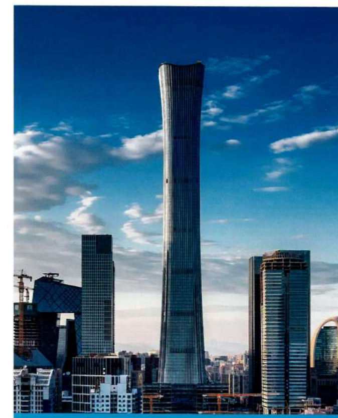
PROJECT: CITIC Tower ARCHITECT: KPF(Kohn Pedersen Fox) PRODUCT: 6 Li+1.52PVB+6 Li Low-E (4 # ) 12A+8C+12A+8C
