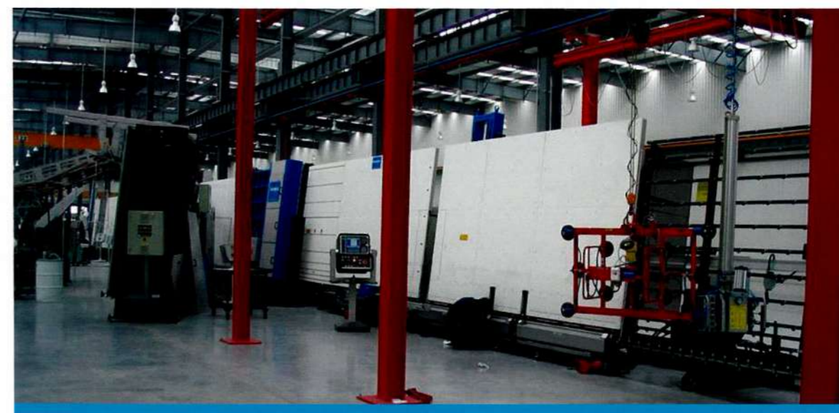
Fully Automated IGU Production Line Manufactured by Germany&Austria
