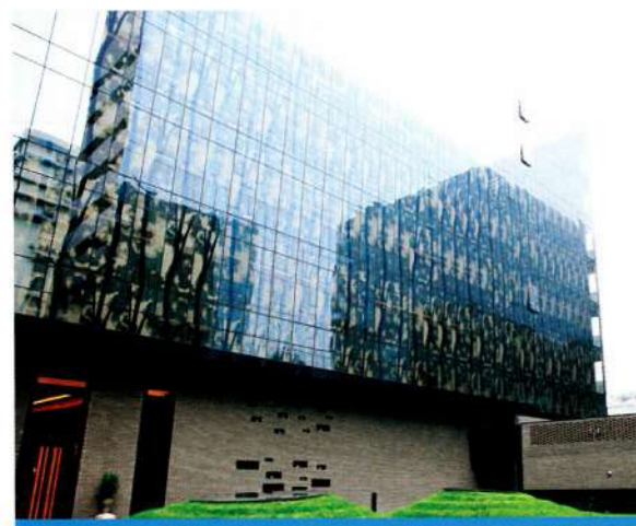
PROJECT: Sino-Ocean Taikoo Li, Chengdu ARCHITECT: The Oval Partnership (Hongkong) MAKE Architects (England) CSWADI(China Southwest Architectural Design and Research Institute Corp.,LTD. PRODUCT: 6YBE0152(2 # ) with frit+12A+6C+1.52PVB+6C
