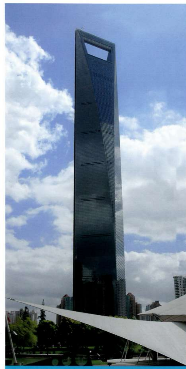
PROJECT: Shanghai World Financial Center ARCHITECT: KPF PRODUCT: 6YSS0116 +0.76PVB+6 C 6 YSS0116+0.76PVB+6C+12A+6C
