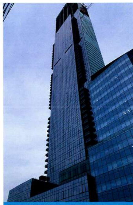
PROJECT: Park view Tower US ARCHITECT: Hill west PRODUCT: 6YRE0646 (2 # )+16Ar+8C 6YTE0670 (2 # )+16Ar+8C
