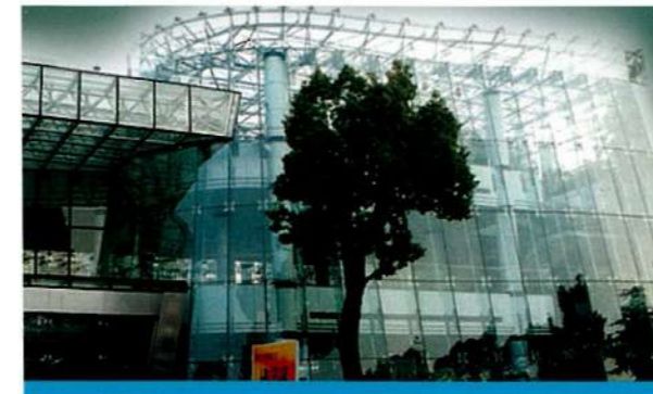
PROJECT: Botanical House of Shanghai People's Garden PRODUCT: 6FT Low-E+1.52PVB+10FT Spider Glass
