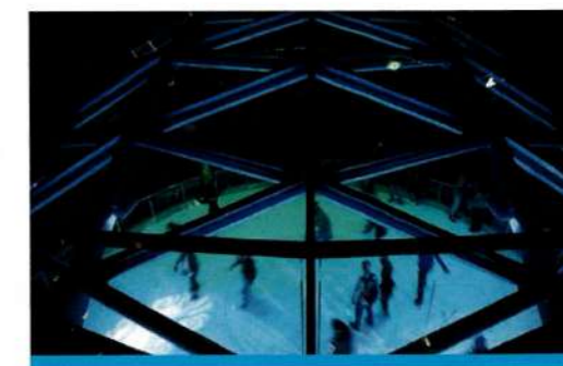
PROJECT : GE PLAZA, Canada PRODUCT :Pilkington Activ™ Clear/Pilkington Energy Advantage™
