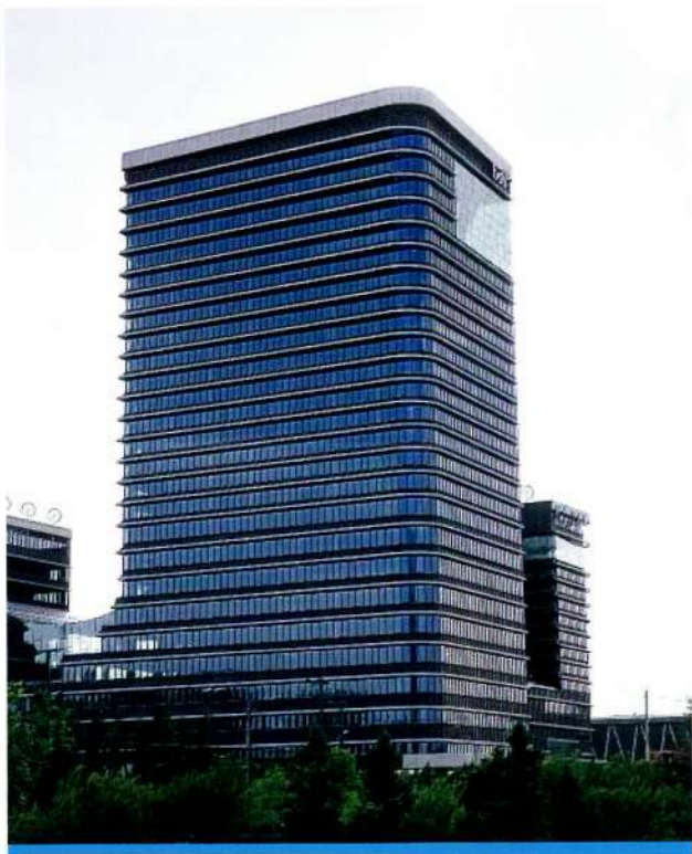
PROJECT: BSB(Baoshang Bank Limited) Plaza ARCHITECT: Beijing Institute of Architectural Design PRODUCT: 8 Li Low-E(2 # ) +12 Ar+8 Crystal Grey+12 Ar+8 Li 8 Li Low-E(2 # ) +12Ar+8 Crystal Grey+12Ar+8 Li (Bend) 12 Li+3.04PVB+12 Li+14 Ar+10 Li Low-E(6 # ) +12Ar+12 Li (Bend)
