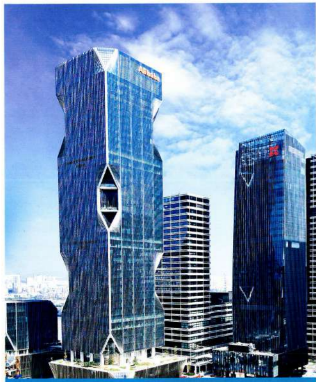
PROJECT: Alibaba South China Operations Center (Guangzhou) ARCHITECT: Guangzhou Design Institute Group CO.LTD PRODUCT: 6C+1.14PVb+6YKE0147(4*)+12A+8C
