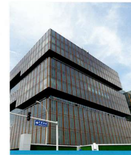
PROJECT: Asian Infrastructure Investment Bank ARCHITECT: Arechitectural Design and Research Institute of Tsinghua University PRODUCT: 10YKE0667T(2 # )+12Ar+10 Li
