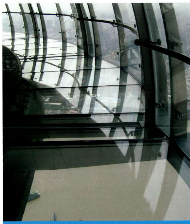
PROJECT: Oriental Pearl TV Tower Hanging Sightseeing Corridor ARCHITECT: Jiang Architects & Engineers (JAE) PRODUCT: 12 Li+2.28SGP+12 Li+2.28SGP+12 Li
