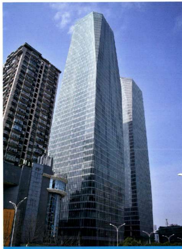
PROJECT: ICC WUHAN ARCHITECT: Woods Bagot PRODUCT: 6 Low-iron+1.14PVB+6 Low-iron with Ultra high performance Low-E coating special for ICC+12A +10 Low-iron+16A+6C+1.52PVB+6C
