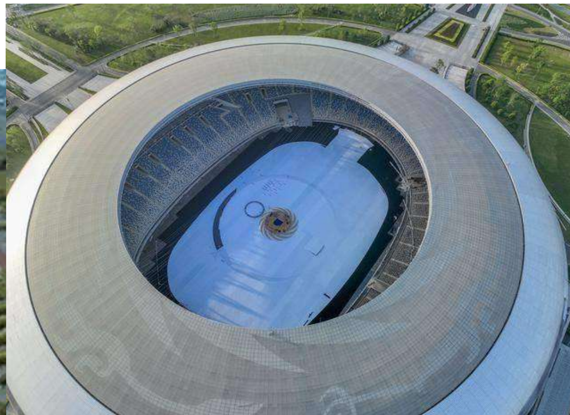
Art Roof with Silkscreen Frit Pattern Glass
