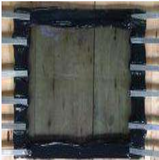
Sealant performance and hardness check
