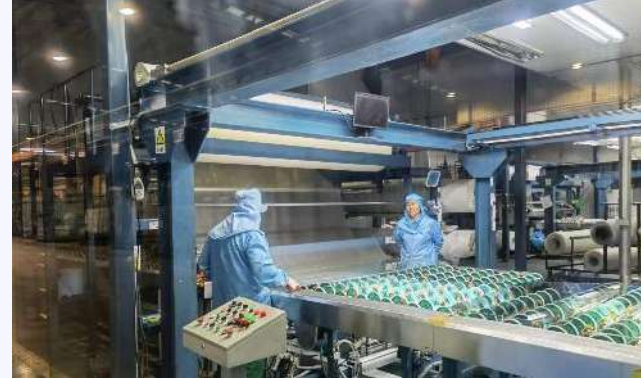
Room temperature, humidity and cleanliness control
